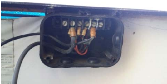
(c). Corrosion
