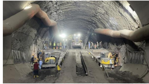
Figure 2. KCIC maintenance machinery equipped with generator and lighting group
