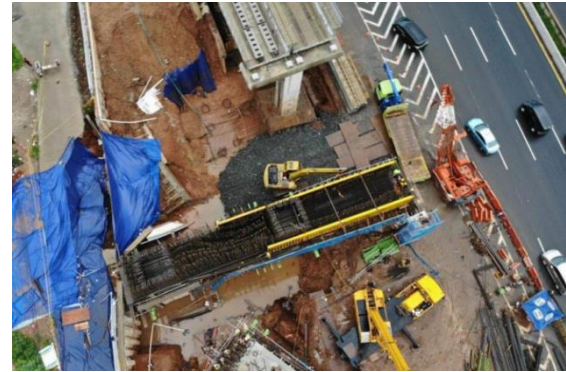
Figure 3. High-speed railway project steps up efforts to deal with extreme weather
